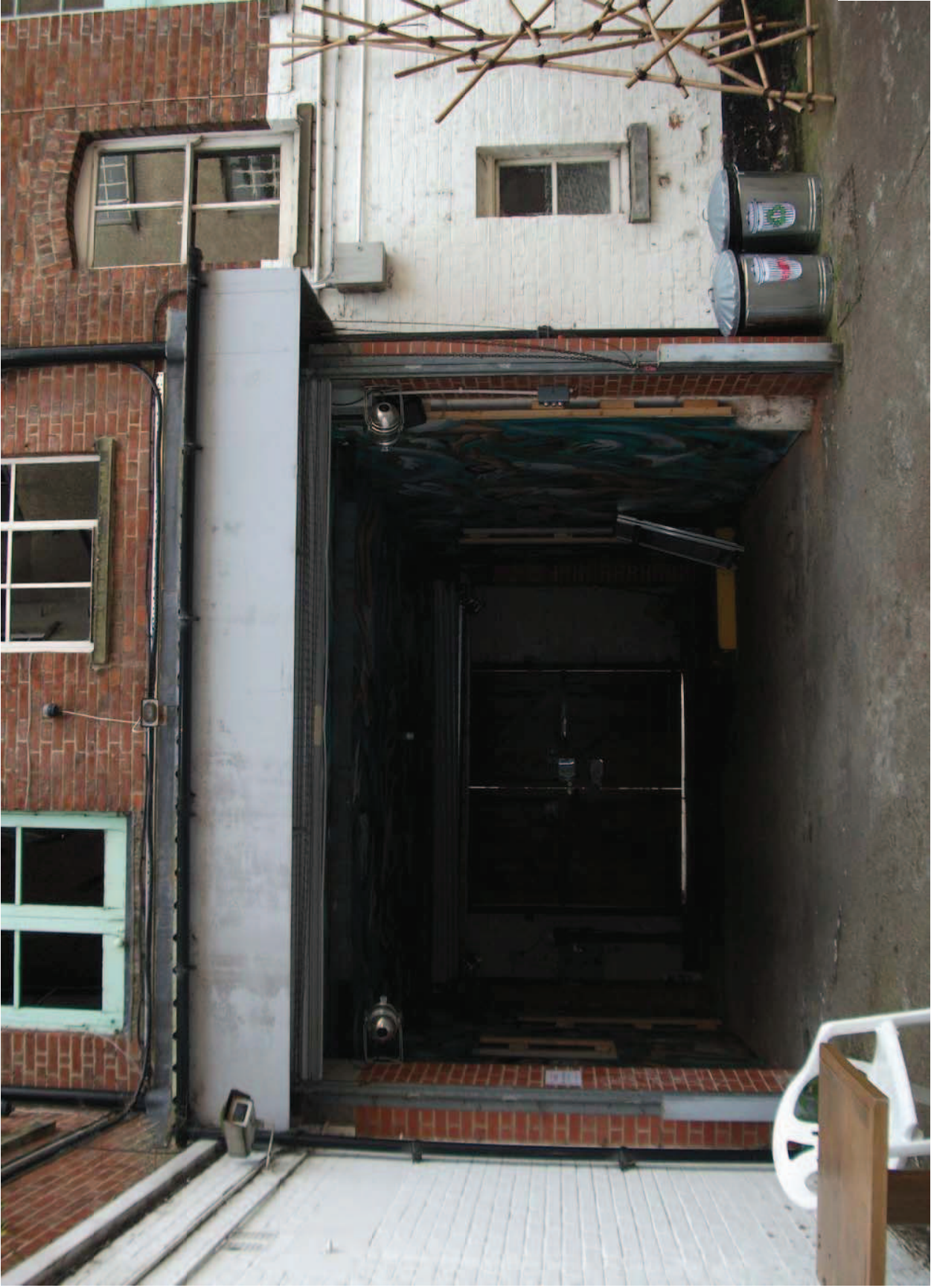
View through to the Pembroke Street entrance
