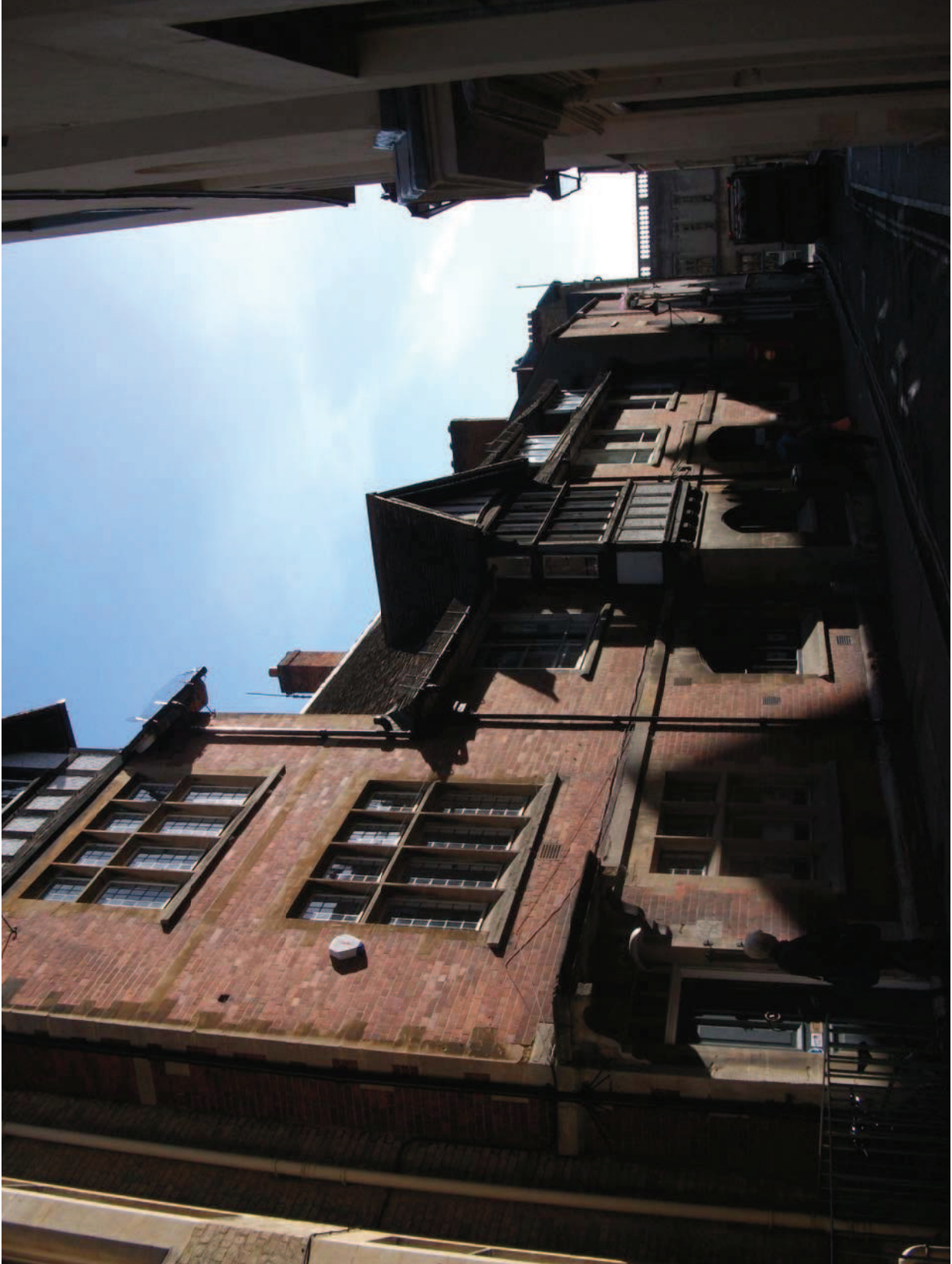
The front elevation of Rochester House, Pembroke Street
